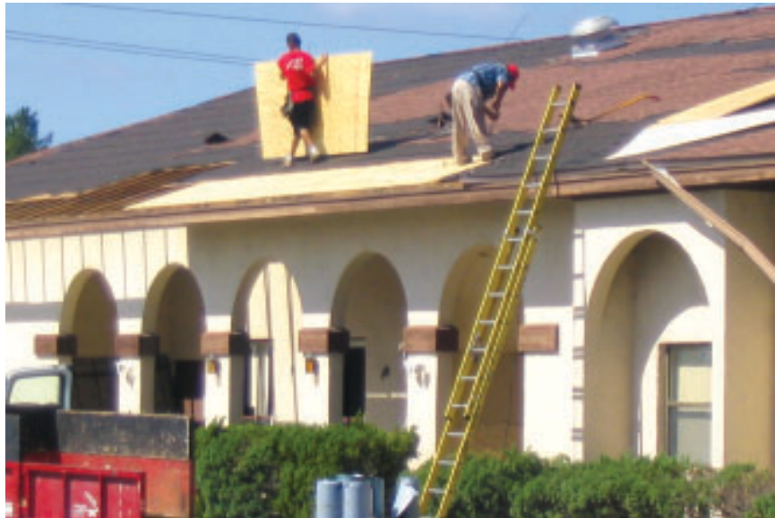
Roofers repair hurricane-damaged facility.
