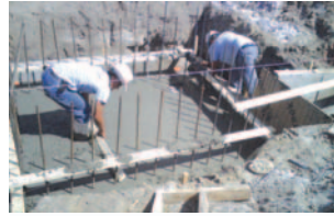
Rising up from the ground...
